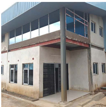
The entrance to the laboratory near completion
