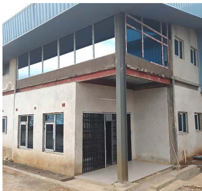
Entrance of the new AISL laboratory near completion
